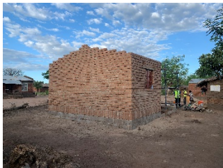
Completing the brick and window and door frame installation
