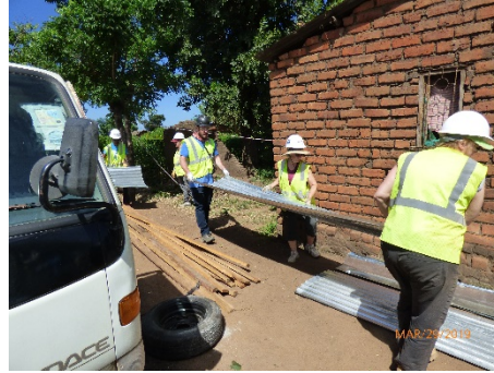
Stacking the roofing galvanized metal sheets
