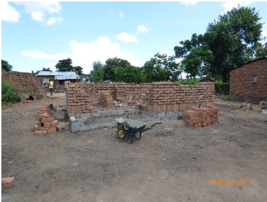
Brickwork beginning. Bricks piled high.
