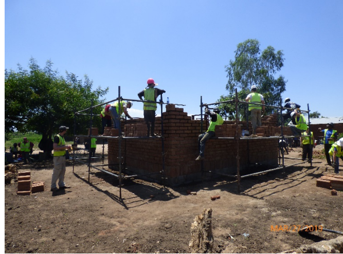
Working from the scaffolding
