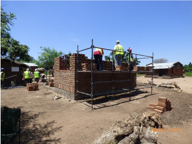
Work continuing on the home – installation of scaffolding.
