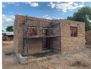
Completing the brick and window and door frame installation
