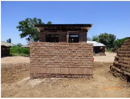
A "work-in-progress" latrine
