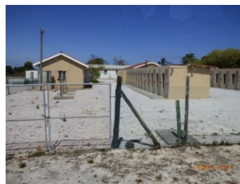
Restored Section of the Jail
