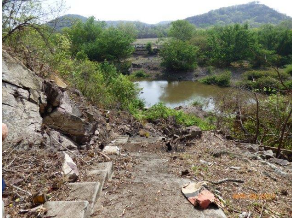
Monte Verde Bridge Site
