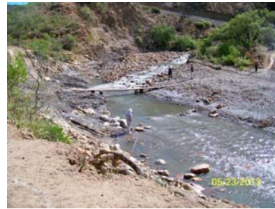
Temporary bridge over the river
