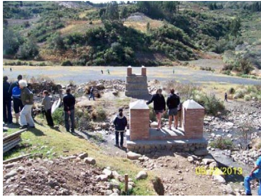
Palca Site – New Bridge in Progress
