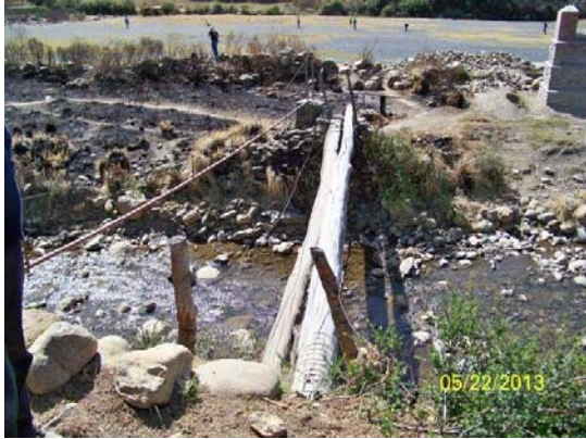
Palca Site – Existing Bridge
