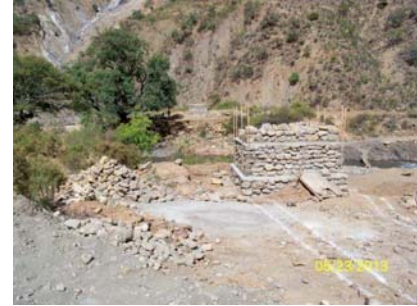
New bridge construction in progress
