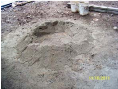
Making the cement
