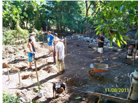
Construction Site at the start of the project
