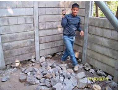
Breaking Rock to Use as Filler
