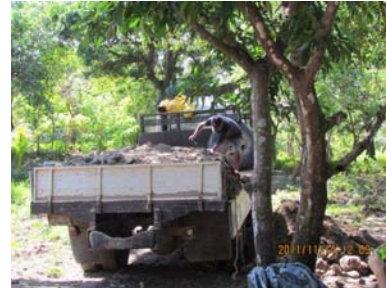
Unloading the dirt - by shovel
