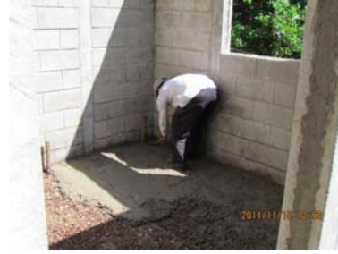
Spreading the rough cement layer
