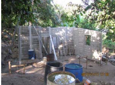
Good Progress - End of Day #4
