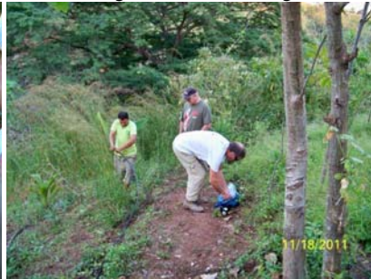
Doug, Jon & Israel installing tubing
