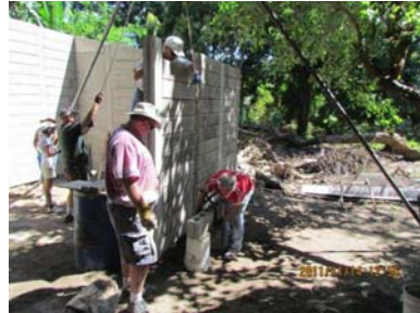
Putting block in place
