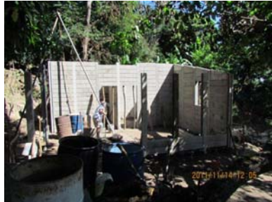
3 columns in place - 2 walls to go.
