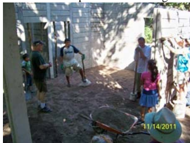
Oscar & Doug - Pounding dirt into place
