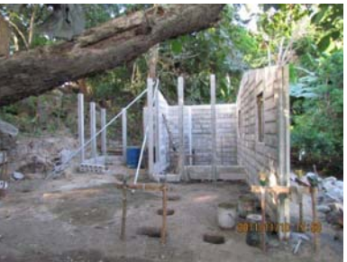
Work Completed - End of Day #3
