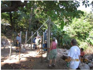
Work in Progress - Day #2
