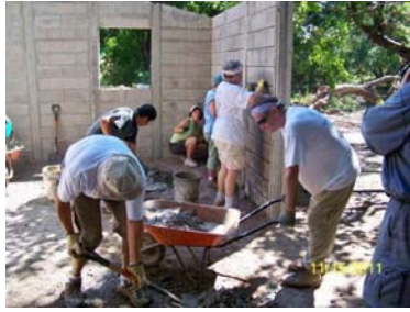
Phase 2 - The rough cement floor
