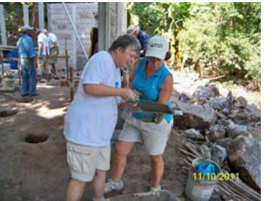
Cement for Pointing Brick
