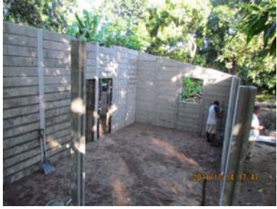
Phase 1 - The dirt floor
