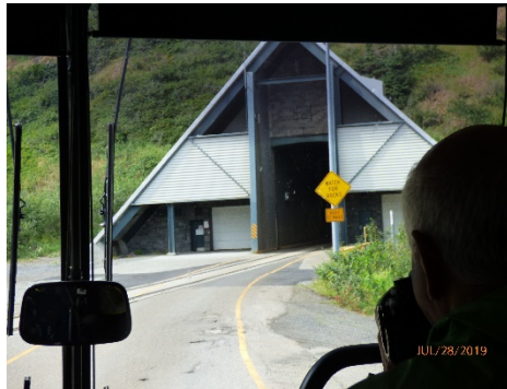
Entrance to Anton Anderson Tunnel
