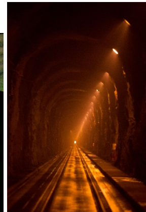
Inside the tunnel
