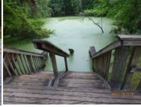
Flooding at the boardwalk
